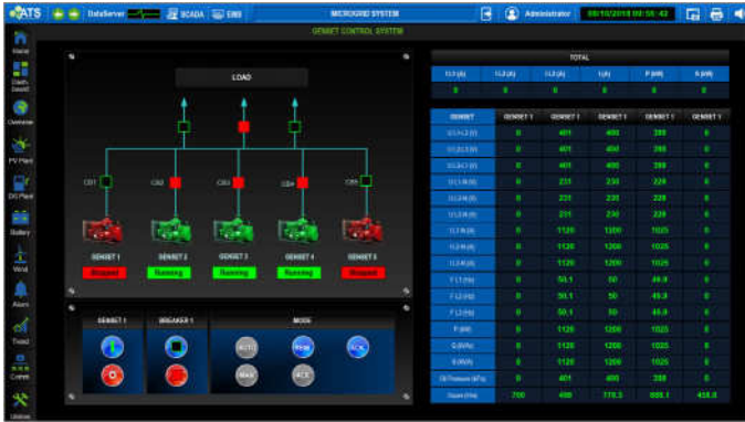
Figure 9. Diesel Generator Overview
