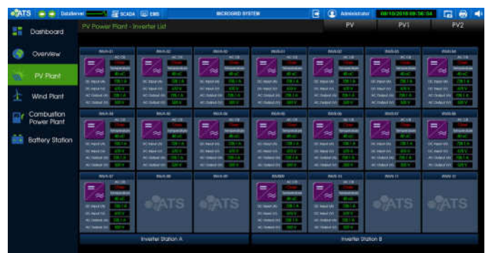
Figure 7. Power Conversion System Monitoring
